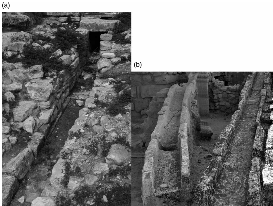
Figure 10 | Minoan sewerage and drainage systems: (a) the output of the central system of the Phaistos palace and (b) part of the central system of the villa Hagia Triada.
